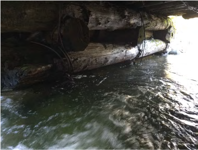
Left Bank Abutment when facing downstream
