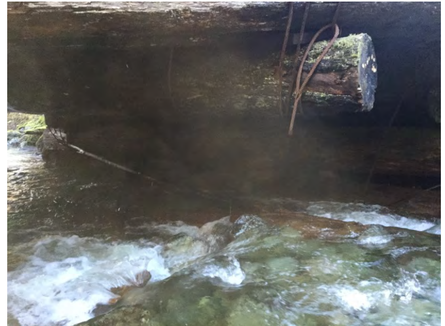
Right Bank Abutment when facing downstream
